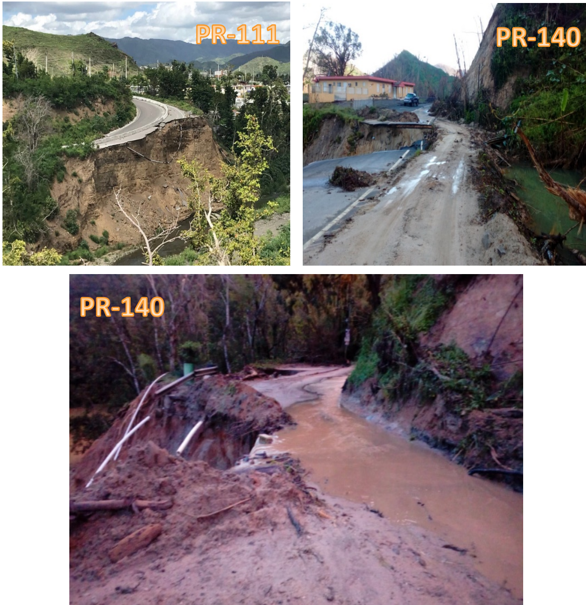
Figure 6.6: Examples Of effects of Hurricane María on the roadway network
