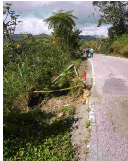
Eroded pavement and landslide Road PR-143 boundary Consejo Ward, Utuado and San Patricio Ward, Ponce
